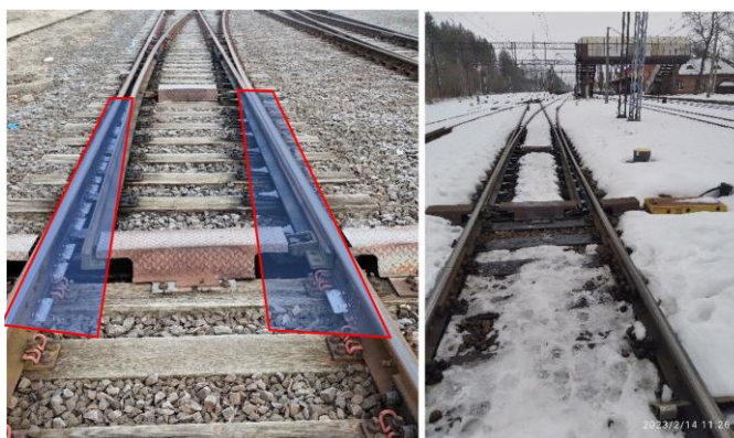
Fig. 1. Heating working area of the stock rails for the right and left half-switch
