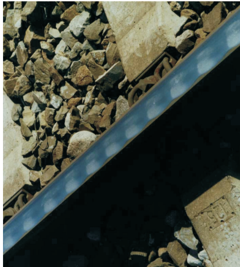
Fig. 1. Wear pattern on the rail head of a narrow curve [1]
