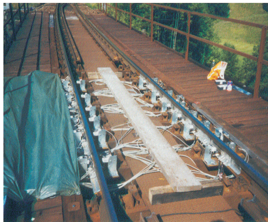
Fig. 6. The measurement site on the steel bridge (without rail corrugations!)
