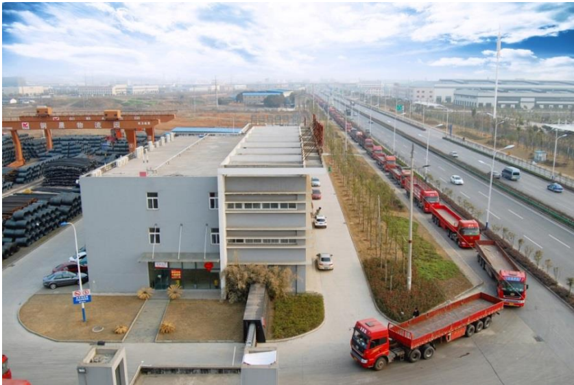
Fig.4. Gangchen Logistics Park View
